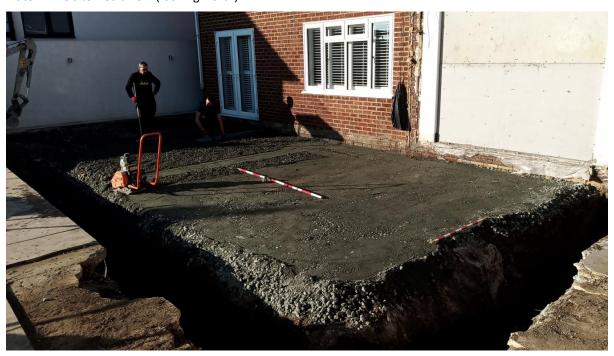
Plate 2. Foundation footings cut and stabilising tarmac surface(looking NW)
